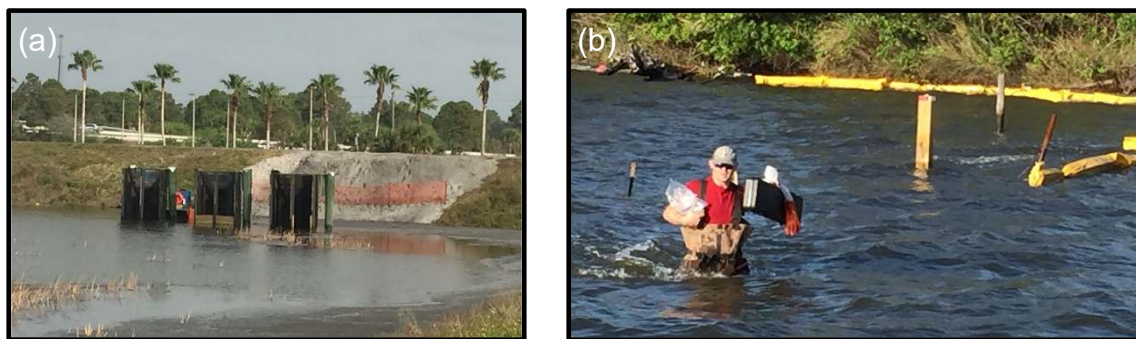
Figure A4. (a) Three weirs in the northeast corner of the DMMA where clarified water flowed over boards into a pipe connected to the IRL and (b) sampling in the IRL along 50- and 100-m radii from the outfall.
