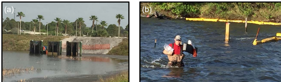
Figure 33. (a) Three weirs located in the northeast corner of the DMMA where clarified water flowed over boards into a pipe to the IRL and (b) sampling in the IRL along 50- and 100-m radii from the outfall.
