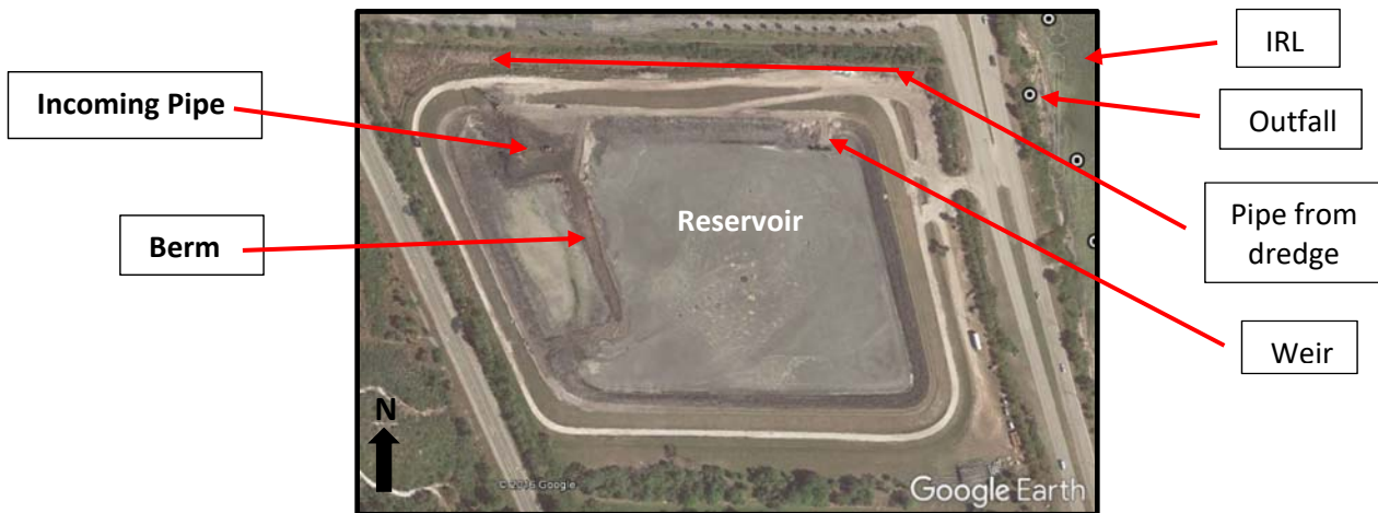
Figure 27. Satellite image of the Palm Bay Dredge Material Management Area (DMMA, BV-52) with arrows and text identifying some of its components and the adjacent Indian River Lagoon (IRL).
