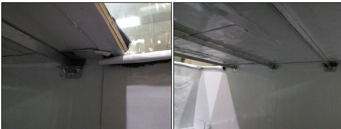
Figure 9: (Left) Overlapping seam-sealers on the inside of the LLB. (Right) The 3 aluminum support bars that keep the lid from bowing under its own weight. The 3 pieces of the lid weigh a total of ~200 lbs.
