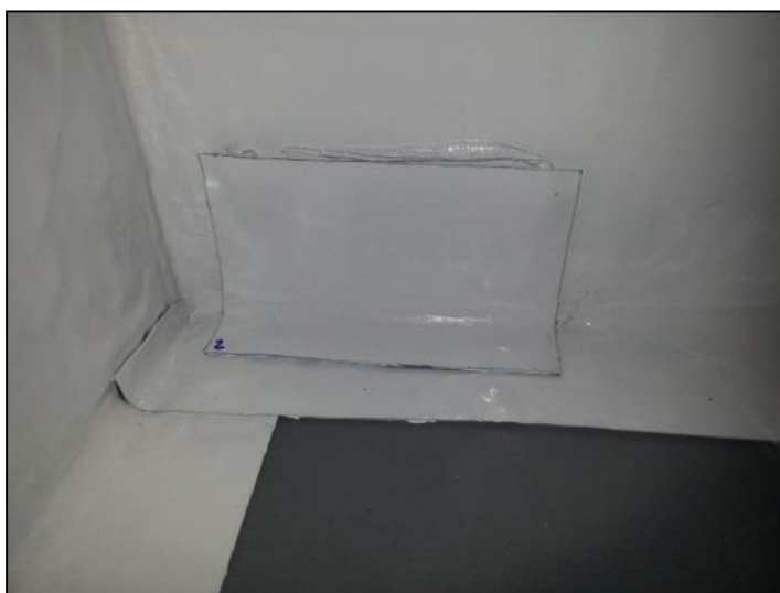
Figure 10: Velcro-attached inside seal of a closed access port. Underneath the solid Velcro-attached seal, but not visible here, is a square 'picture frame' seam-sealer that is permanently glued around the cut in the large side panel's lead.
