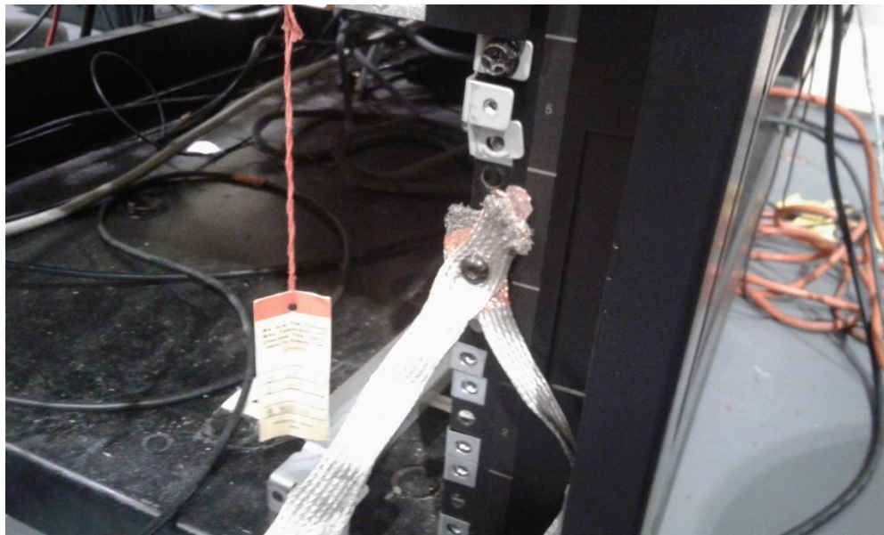
Figure 8. Image of Ground Straps Connected to MHEP Rack 1
