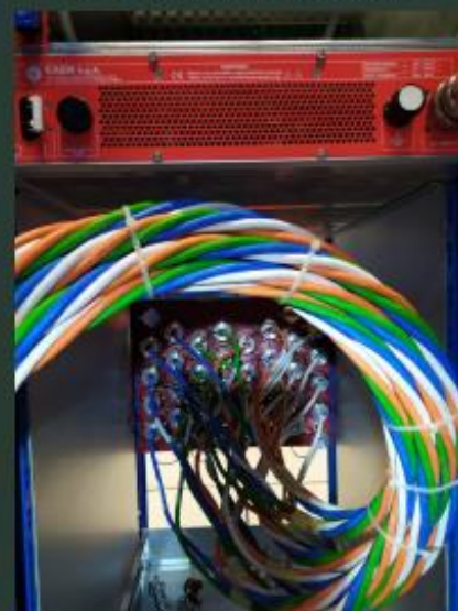
USC rack front side
