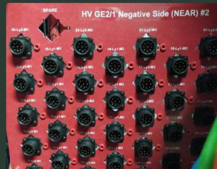
USC Patch panel front side
