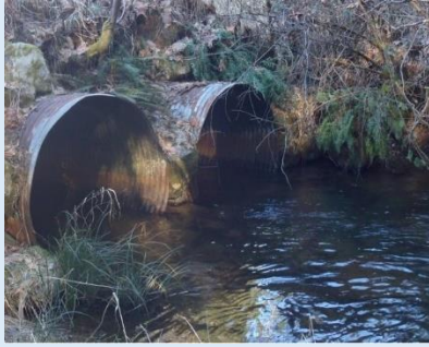
These barrier culverts on Bush Creek near Elma have been replaced, opening 8.2 miles of forested habitat for fish.
