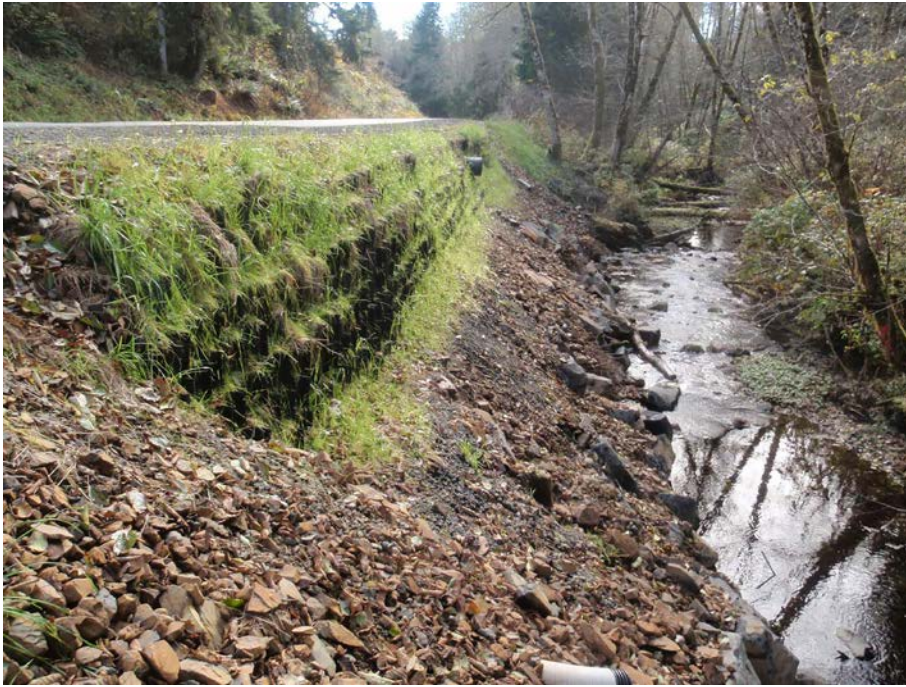
Vegetated MSE slope. Credit: ODOT
