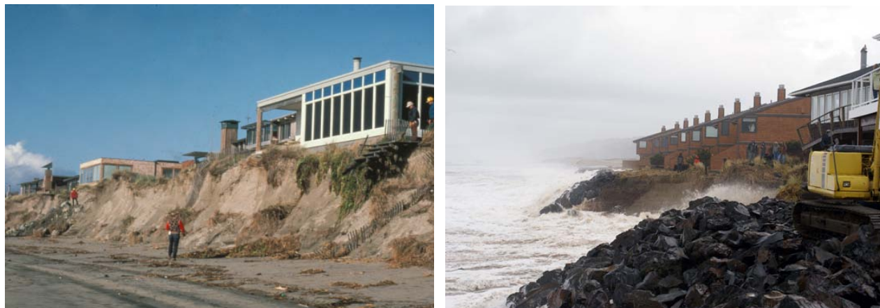
FIGURE 6.9 Construction of private homes on the frontal dunes. (Left) Homes in central Monterey Bay were threatened by erosion during the high tides, elevated sea levels, and large storm wave of the 1983 El Niño. SOURCE: Courtesy of Gary Griggs, University of California, Santa Cruz. (Right) Placement of riprap during storm conditions to protect development on dunes in Neskowin, Oregon. SOURCE: Courtesy of Armand Thibault.
