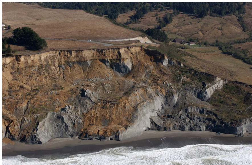
FIGURE 6.2 Large-scale landsliding along the Humboldt County, California, coast at Centerville. SOURCE: Copyright 2002-2012 Kenneth & Gabrielle Adelman, California Coastal Records Project, < www.Californiacoastline.org >.
