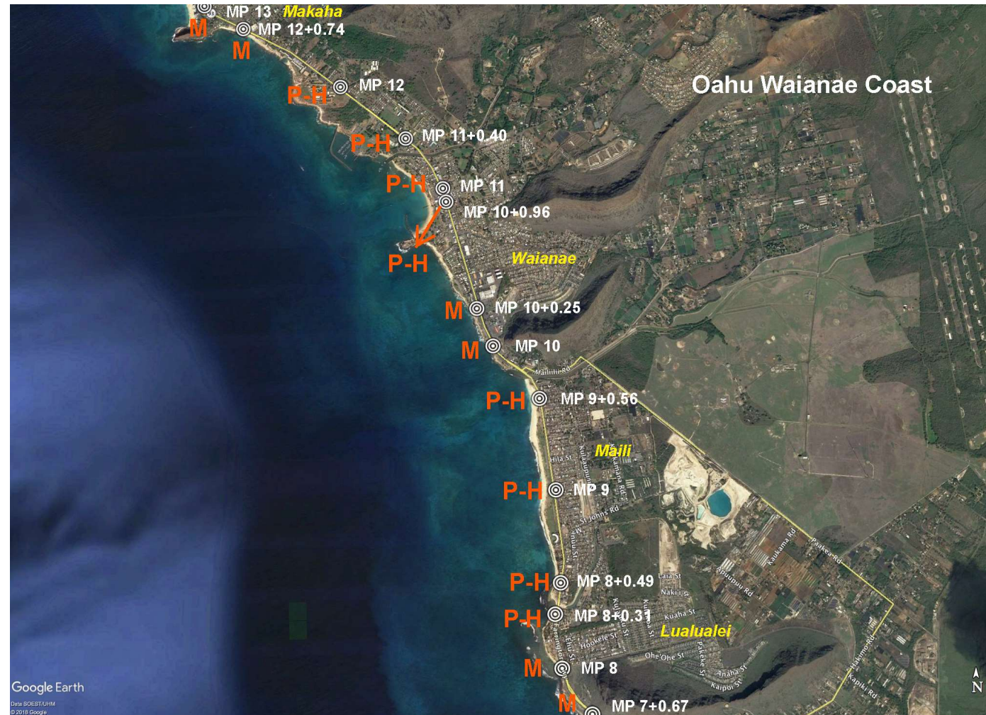
Figure 4.7. Lualualei to Makaha adaptation recommendations for the State of Hawaii Statewide Coastal Highway Program Report (for table version, see Table 4.2). R-N is road relocation to new road; P-SD is living dunes; P-H is hard protection; C-H-E is elevate/hard protection; C-H-SD is hard/soft protection; M is no action/monitor.
