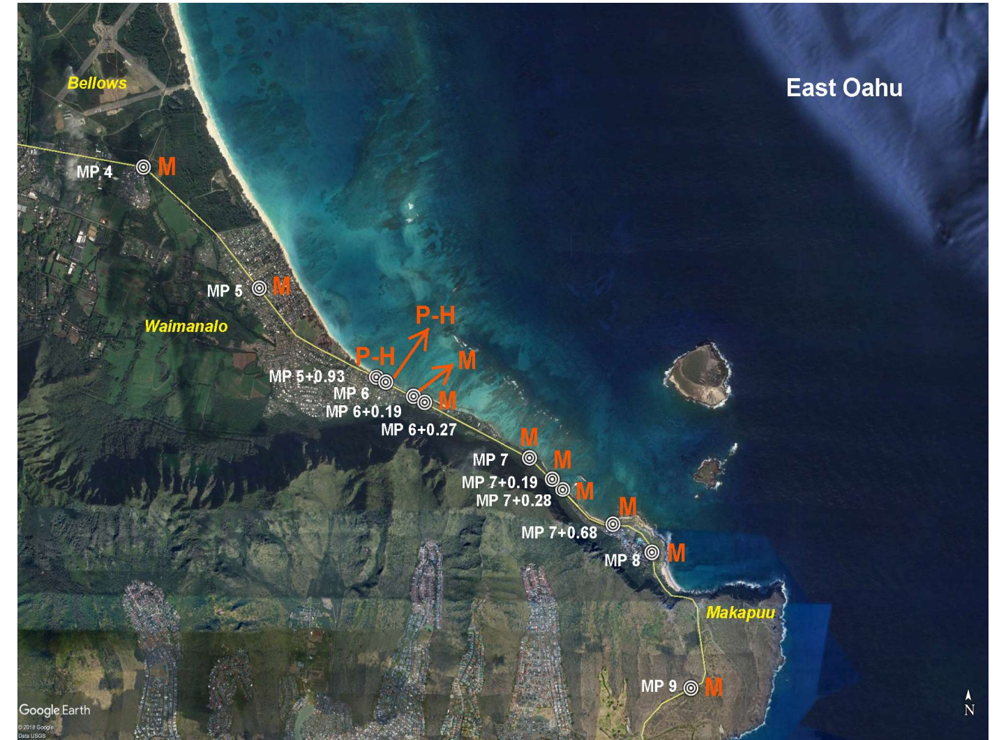
Figure 4.4. Waimanalo to Makapuu adaptation recommendations for the State of Hawaii Statewide Coastal Highway Program Report (for table version, see Table 4.2). R-N is road relocation to new road; P-SD is living dunes; P-H is hard protection; C-H-E is elevate/hard protection; C-H-SD is hard/soft protection; M is no action/monitor.
