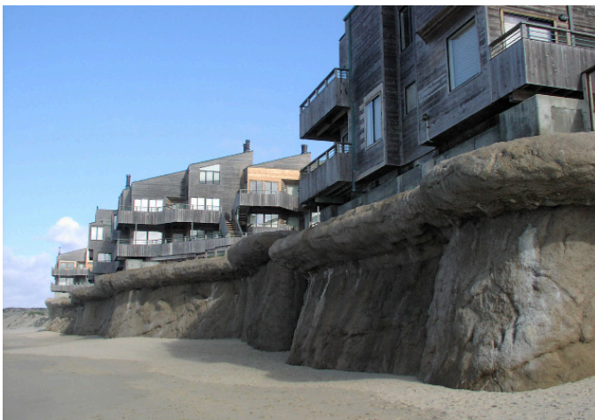
Figure 5.1. Ocean Harbor House condominiums in Monterey were built too close to an eroding dune face, which ultimately led to the construction of a massive concrete seawall for protection.
