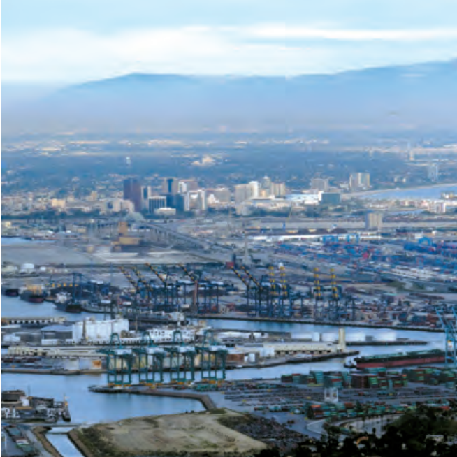
New decision-support tools that incorporate sea-level rise into investment decisions for upgrading coastal infrastructure are vital to California's economy.
