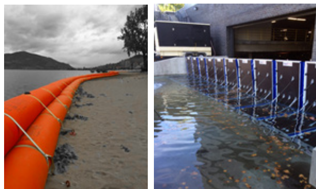
Figure 19: Examples of temporary flood barriers: Tiger Dam (left) and Aquafence (right)
