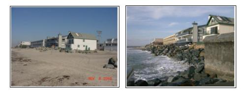
**Figure 3.** Impact of coastal armoring on public beach—with sand following nourishment (**left**), and without sand (**right**). Photo: J. Nakagawa.
