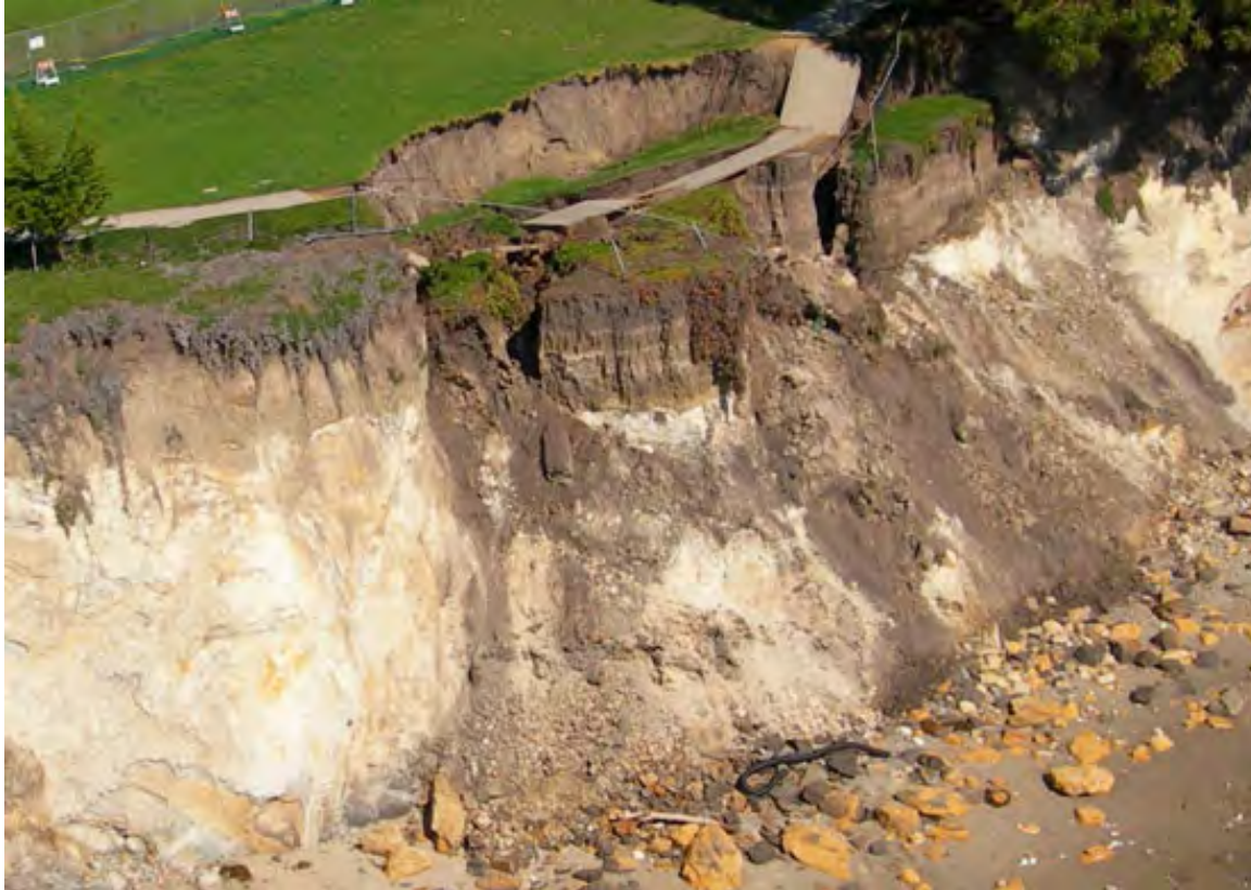
Figure 2.7: January 2008 Landslide along the Cliff at Shoreline Park Moved the Cliff Edge Landward by as Much as 38 Feet and Eliminated a Portion of the Sidewalk
