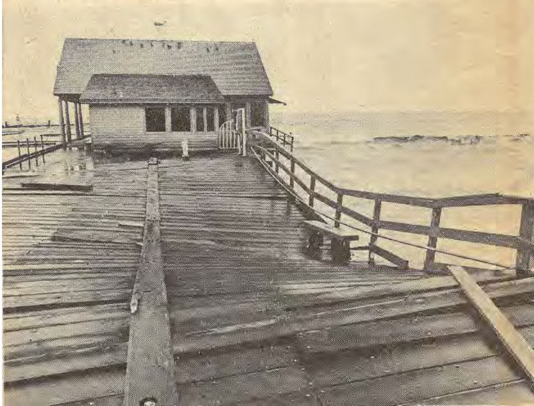
Figure 2.16: The End of Stearns Wharf Sags from a Loss of Pilings in early March 1983 Due to Impacts of Large Waves at Times of High Tides and Elevated Sea Level
