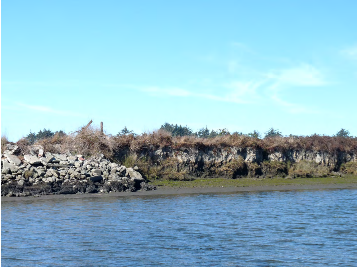
Figure 25. Mad River Slough is an example of contrasting shorelines one that is exposed and the other with concrete revetment on Humboldt Bay.
