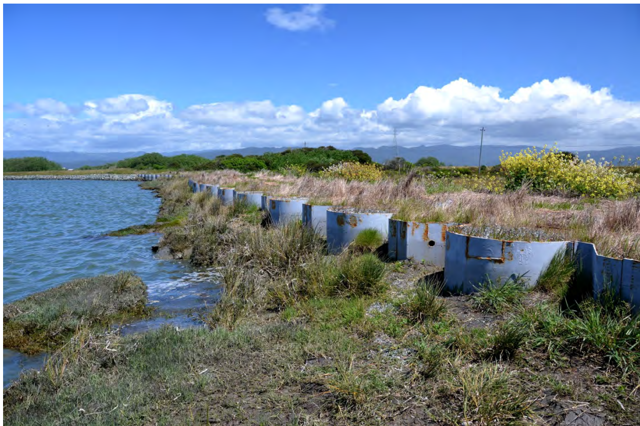
Figure 29. Mad River Slough is an example of a shoreline that is covered by a steel bulwark on Humboldt Bay.
