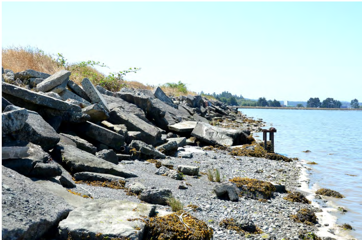
Figure 27. Arcata Bay is an example of a shoreline that is covered with concrete revetment on Humboldt Bay.
