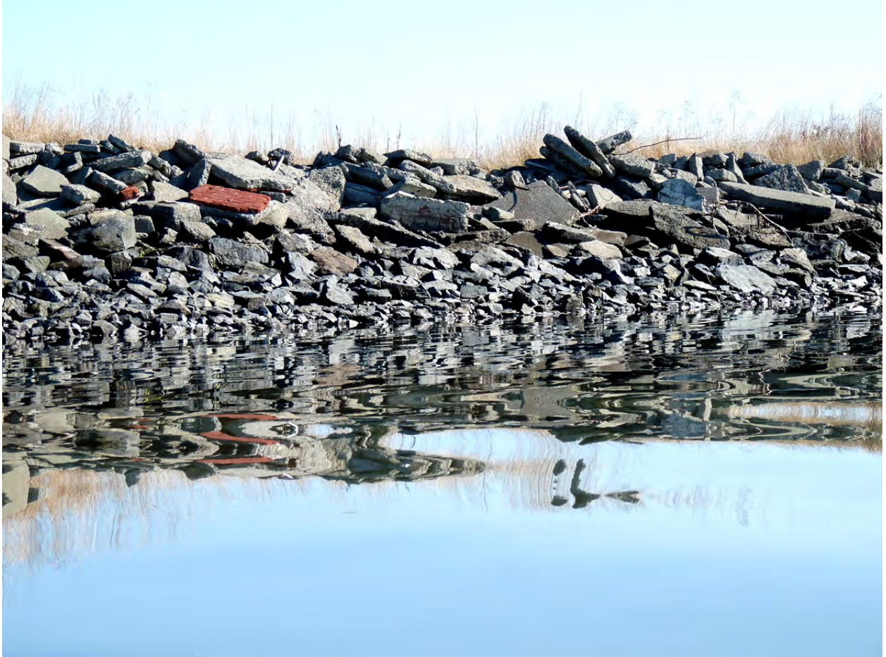
Figure 30. Arcata Bay is an example of a shoreline that is covered by a rock and concrete revetment on Humboldt Bay.
