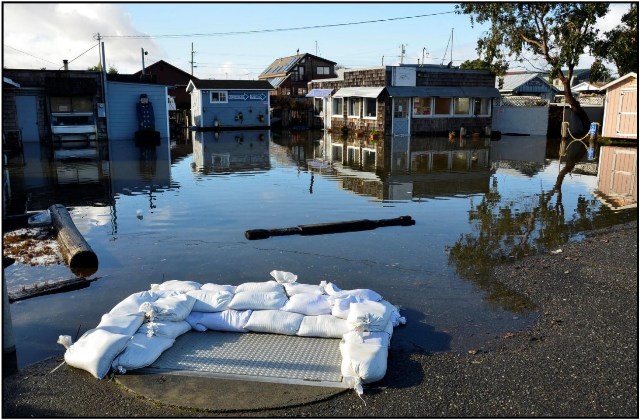
Figure 26: Sandbags on King Salmon Drive to protect stormwater infrastructure (Laird 2018).
