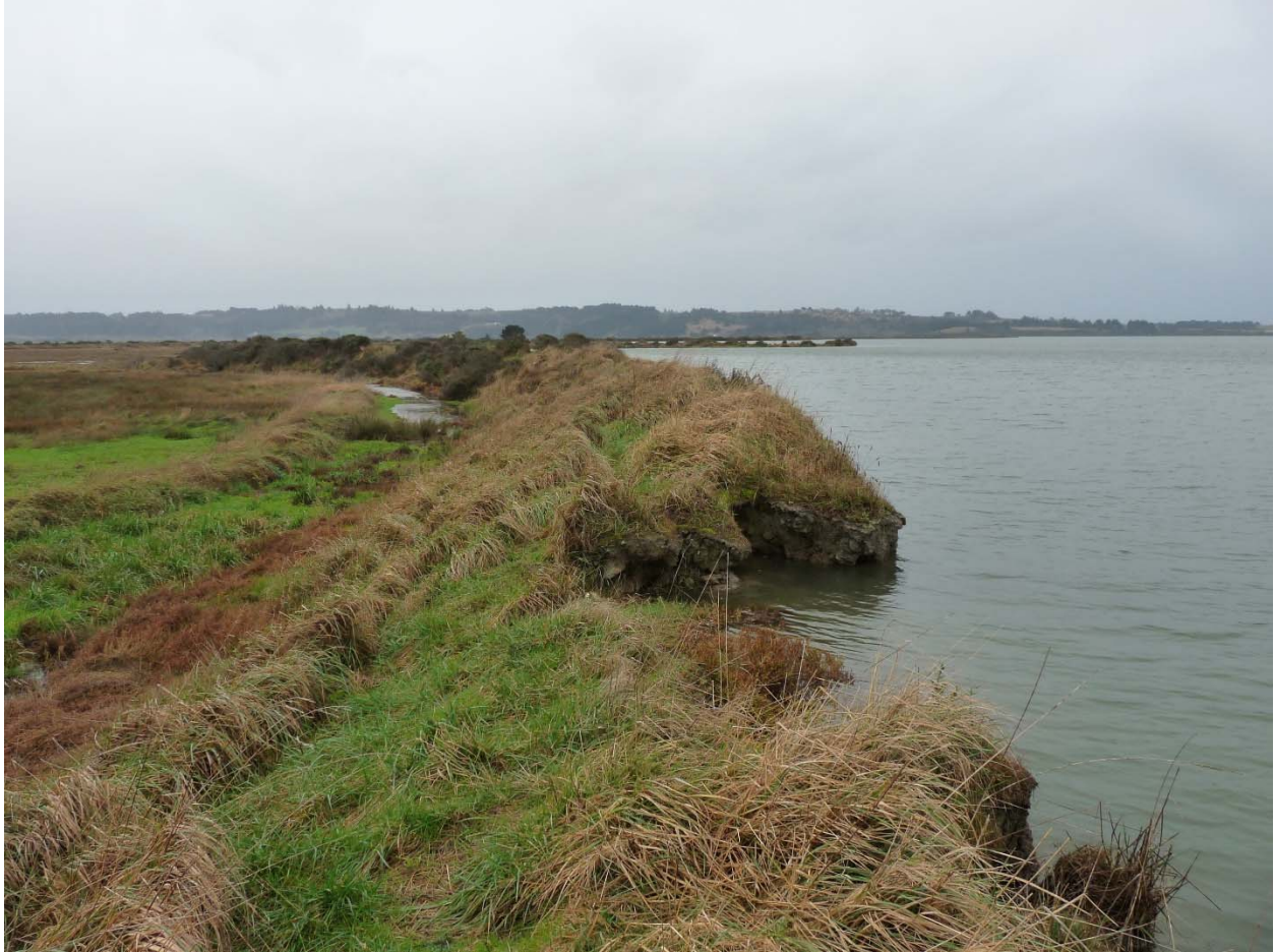
Figure 8. Eroded and low elevation dike shorelines are vulnerable to breaching during King tides and/or storm surges.
