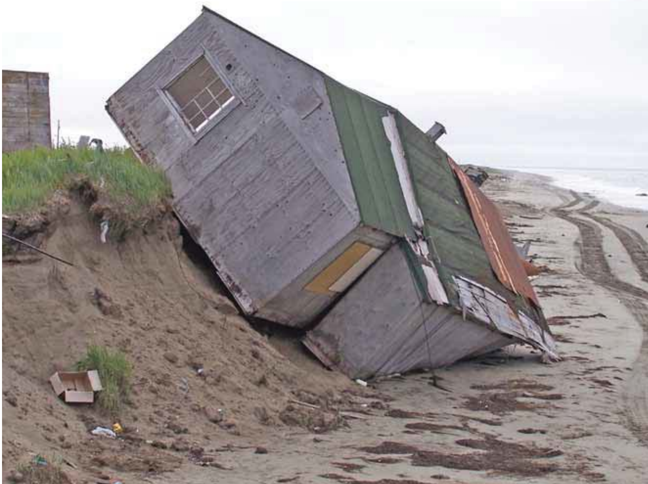
Figure 18. Rapid erosion during fall storm events has resulted in collapse of several structures in the coastal community of Shismaref, near BELA.
