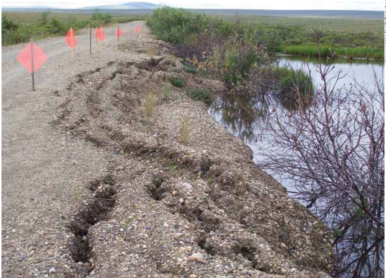
Figure 23. Thermokarst formation and road collapse on the Nome to Taylor Highway, outside of Bering Land Bridge (BELA). The pond resulted from thawing and collapse of ground ice.
