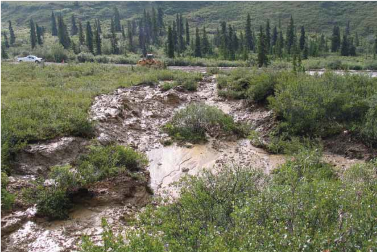
Figure 24. Quick responses were necessary when active layer thaw and collapse resulted in mudflows blocking the Denali Park Road.
