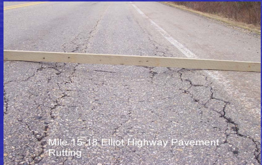
Alaska Highway Damage and rutting
