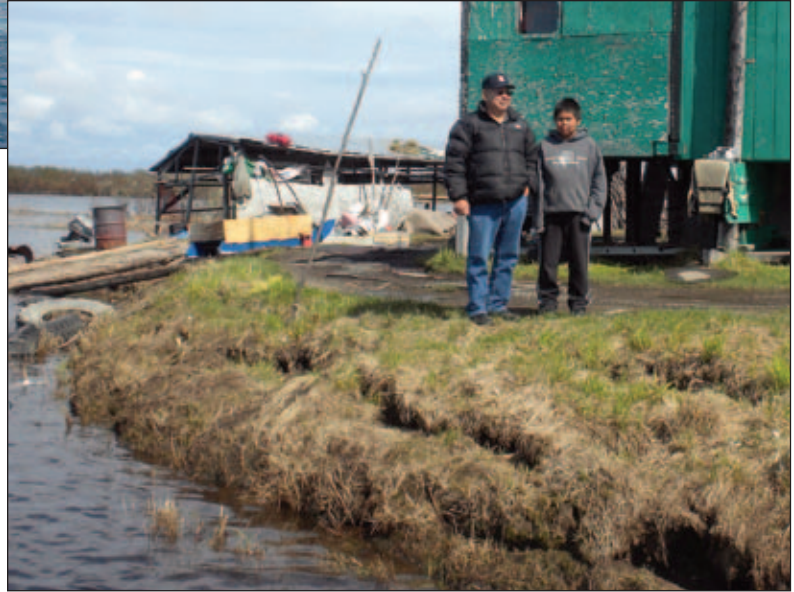
The home of Daniel Foster Sr. is one of many threatened by bank erosion. Mike Brubaker, 2011.
