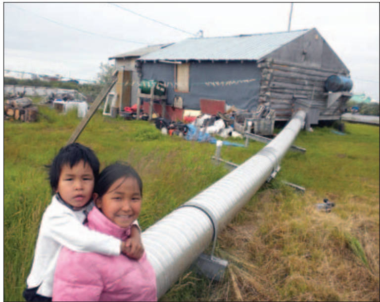
The Snyder kids are all smiles despite the sagging Arctic pipe that brings water to their home. Mike Brubaker, 2011.
