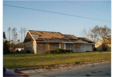
The loss of roof cover and underlayment can lead to significant water intrusion.
