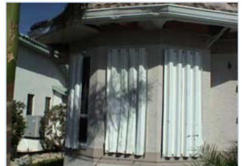
These shutters took a beating from roof tiles that were blown off a neighboring house, but still managed to protect the openings.
