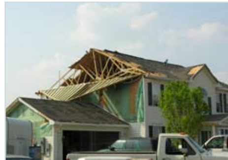
Gable end wall and roof sheathing damage.
