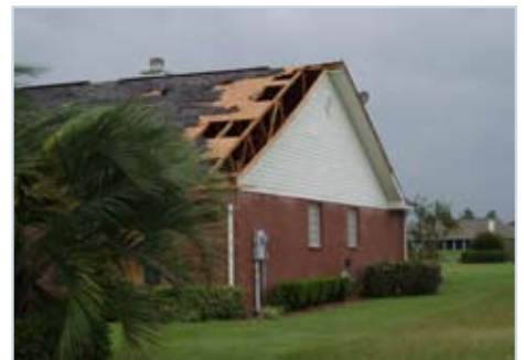
Loss of roof sheathing allows water and wind inside.
