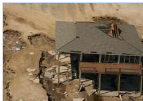
Figure 22 Aerial photos taken after Ike showed close to 90 percent of the homes near the coast toward the western part of Bolivar Peninsula had an extensive loss of hip and ridge shingles.
