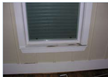
Figure 38 Water got inside this window, despite the presence of a hurricane shutter and the use of impact-resistant glass.
