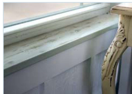
Figure 37 Even during a Category 2 hurricane, where rainfall rates never exceeded a rate of about 1 inch per hour, wind-driven rain leaked into the house through windows and doors.
