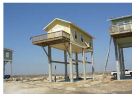
Figure 31 While all of the decks did break away, it is clear that deck connections were not what typically would be considered a breakaway connection in the Coastal Construction Guidance from FEMA and the NFIP.
