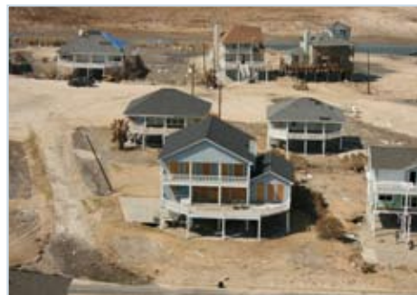
Figure 22 Aerial photos taken after Ike showed close to 90 percent of the homes near the coast toward the western part of Bolivar Peninsula had an extensive loss of hip and ridge shingles.
