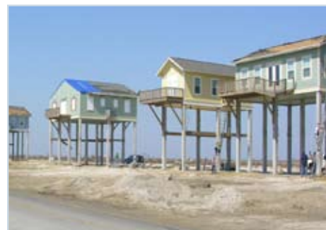
Figures 29 and 30 Ground level views, looking west, of the Fortified houses before and after Hurricane Ike. It is clear that all storage areas and decks were totally destroyed by the storm surge.
