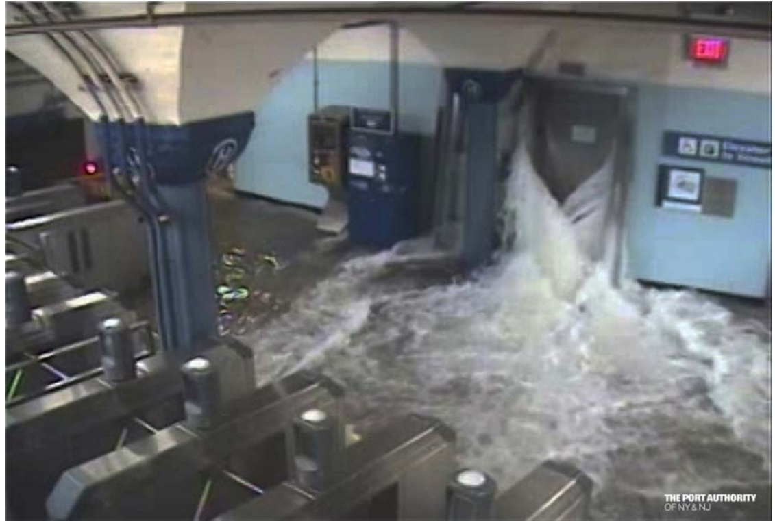
FIGURE 3.2 During super storm Sandy in 2012, storm surges brought water inland and flooded subway terminals in the New York area—part of the billions of dollars in damages from that storm. SOURCE: Port Authority of New York and New Jersey.
