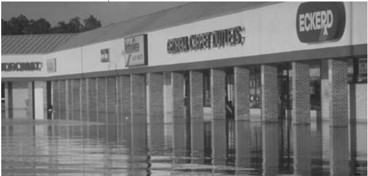
Strip mall closed in Albany, Georgia after floodwaters reach waist high. Photo: U.S. Army Corps of Engineers
