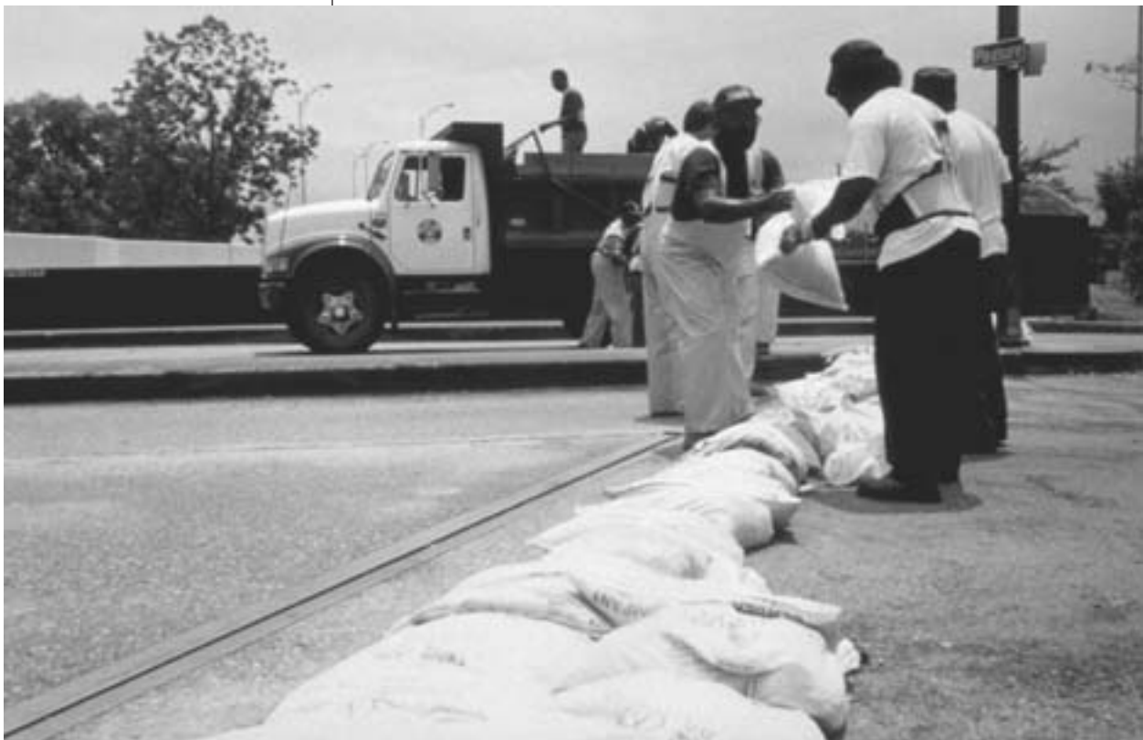
Sandbagging in New Orleans, May 1995. Photo: U.S. Army Corps of Engineers
