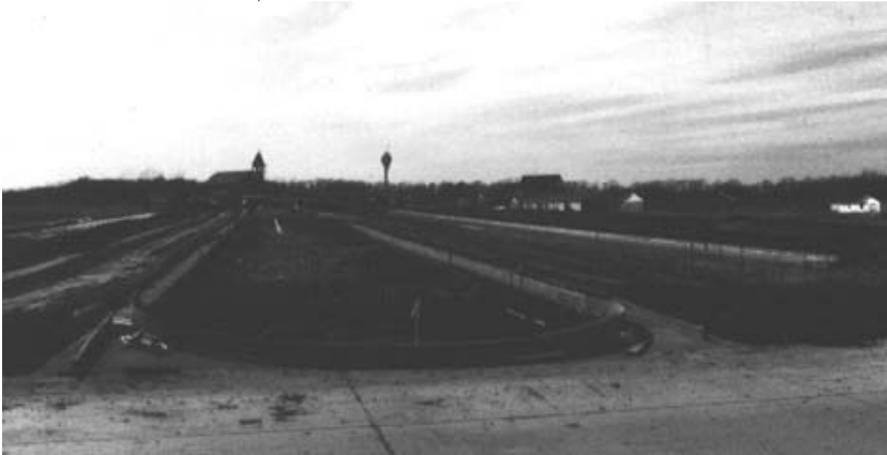
New Valmeyer, Illinois under construction. After the 1993 Midwest Flood, residents of Valmeyer decided to move their town off the Mississippi bottoms to higher ground. Photo: Illinois Department of Natural Resources
