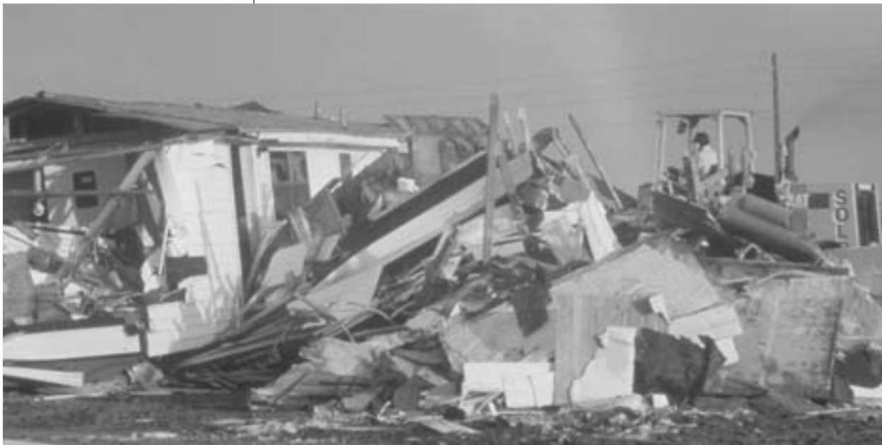
Bulldozer removes mobile home in Perrine, Florida. Photo: NOAA
