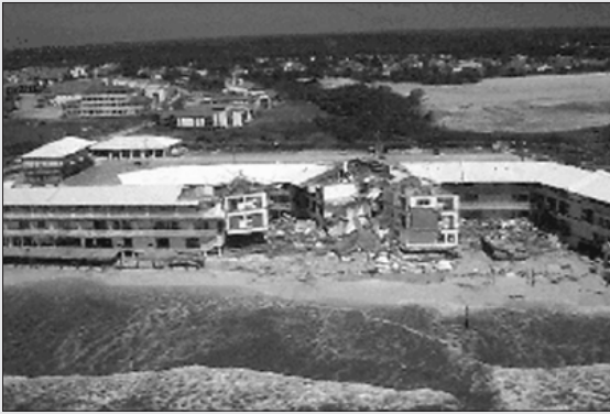
Destruction along the Gulf Coast of Florida, October 1995.
