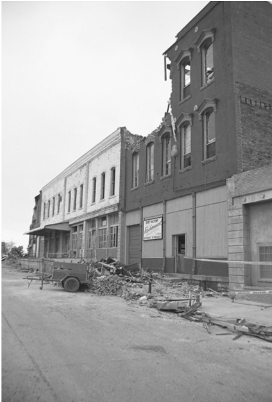
Figure 4.3 Many homes and businesses suffered extensive damage from Hurricane Andrew, one of the most destructive hurricanes ever recorded in the United States. Source: FEMA News Photo.
