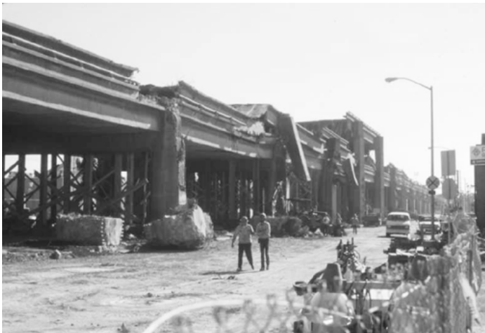
Figure 2.3 The Cypress Street section of Interstate 880 collapsed in Oakland, California, following the Loma Prieta earthquake. Photo by S. Cutter.
