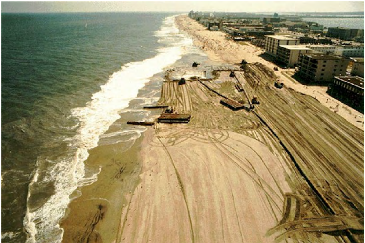
FIGURE 1-10 Beach nourishment in Ocean City, New Jersey.
