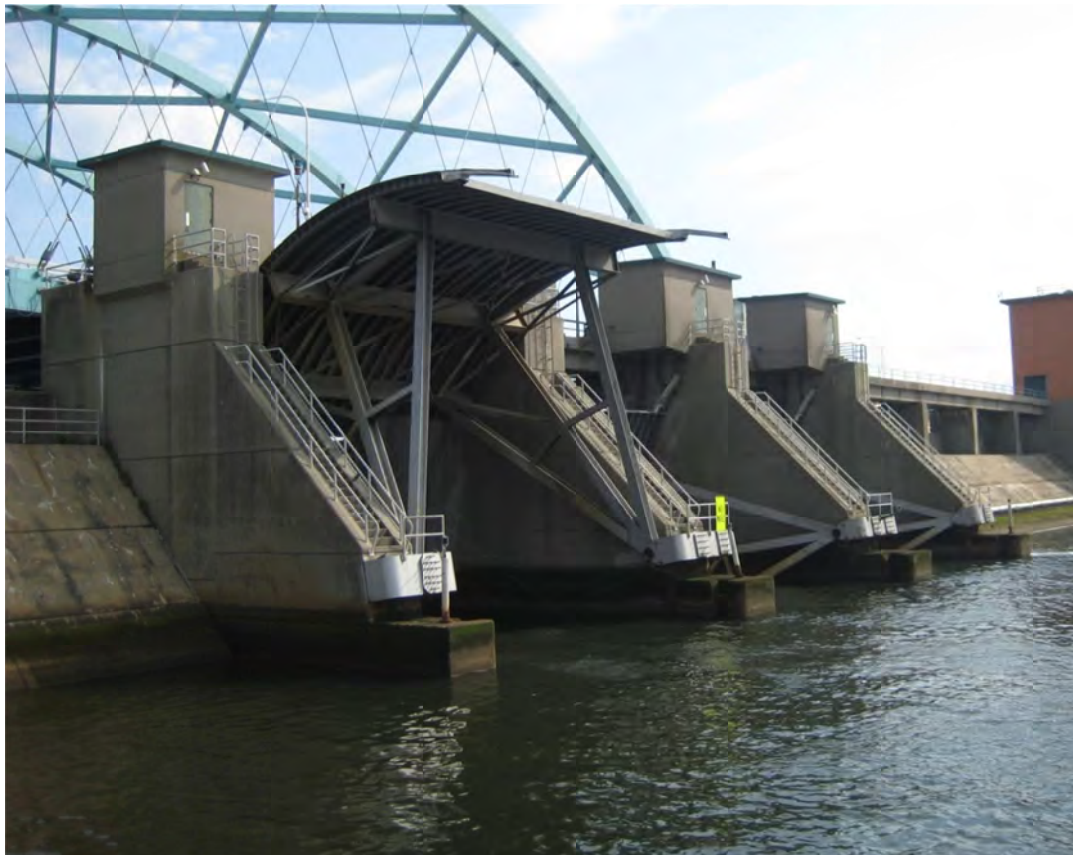
FIGURE 1-8 Fox Point hurricane barrier on the Providence River in Providence, Rhode Island, built in 1966.
