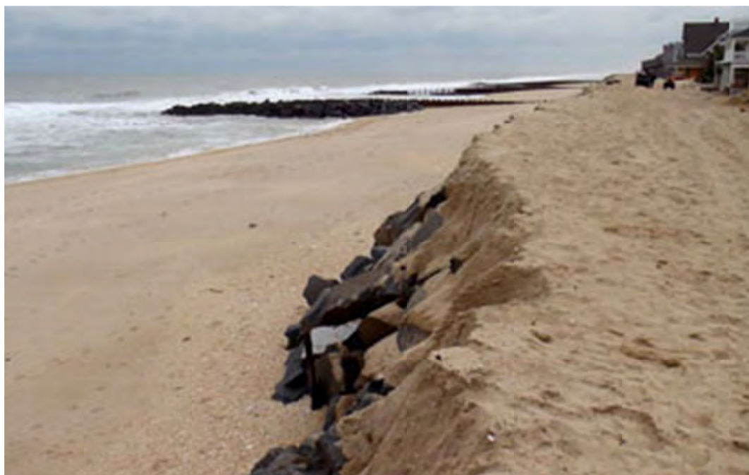
FIGURE 3-4 Relic seawall in Bay Head, New Jersey, that was buried beneath a dune and uncovered during Hurricane Sandy.
