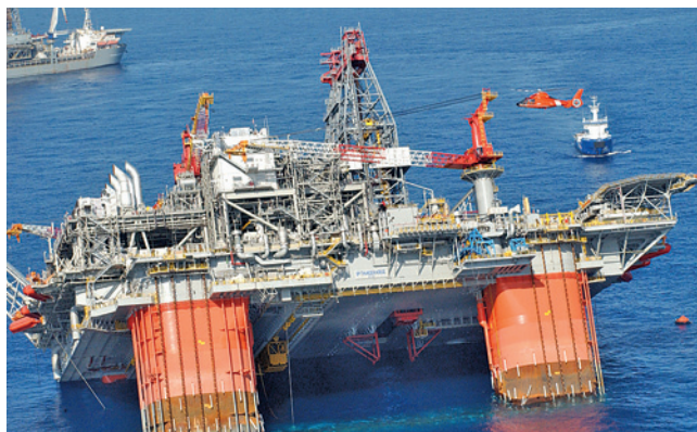
FIGURE 17: Hurricane damage to the Thunder Horse platform.
