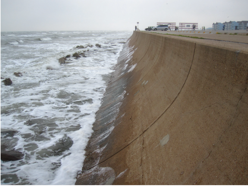
FIGURE 1-6 Seawall along the coast of Galveston Island, Texas.
