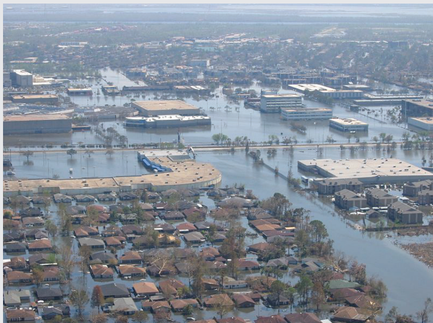
FIGURE 1-4-1 Flooding of New Orleans after Hurricane Katrina.
