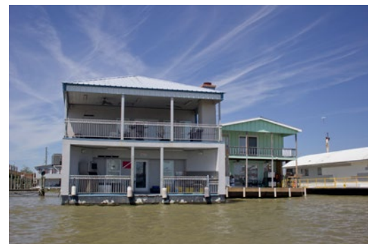
Figure 66. Historic Building Methods
