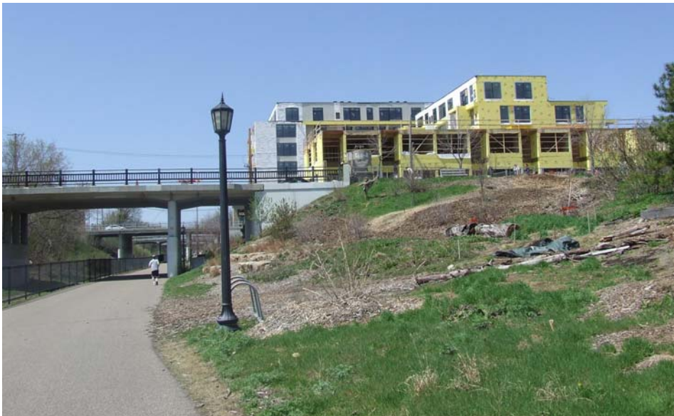
Figure 2. Midtown Greenway (Minneapolis, MN).
