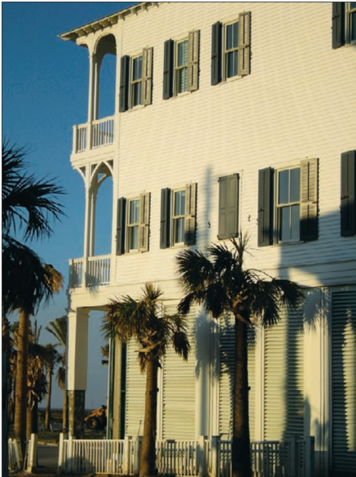
Figure 8-6. Beachtown, TX, under construction
