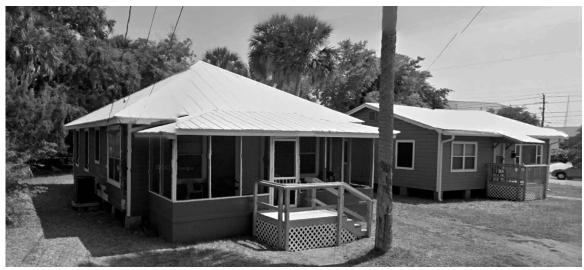
Fig. 35: Vernacular frame houses in the Lincolnville district were originally constructed on block piers, some coquina. The added height currently protects from repetitive flooding in the area. This area on Duero Street, the district's western border, is likely to be flooded by 2100. [Google Earth; street view photograph, 2013]
