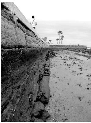
Fig. 40: Part of the nineteenth century seawall borders the Castillo. At low tide, the deterioration from wave action and dissolution is evident on the coquina wall. [Ann Horowitz; photograph, January 2013]
