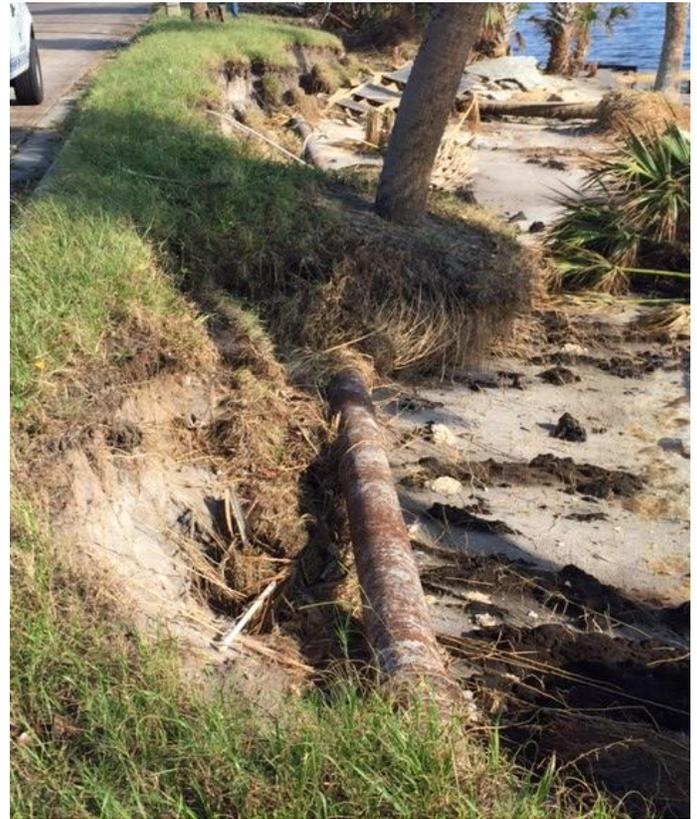
*This image shows how erosion and flooding can begin to impair the integrity of roadways long before inundation occurs and also cause damage the underground utilities.*
