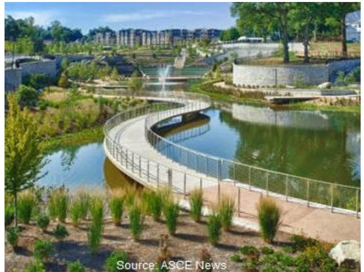
*The image shows “Fourth Ward Park” in Atlanta, Georgia, a great example of this park concept. In this park, walkways traverse through stormwater ponds and native plants are used to absorb rainwater without diverting it into drains.*
