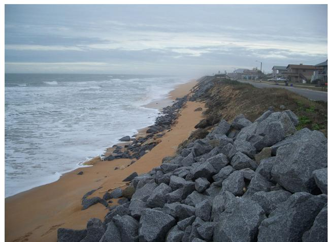
**Fig. 2** Failing rock revetment at South 17th Street, Flagler Beach, Florida. Author’s Photo, January 2014
