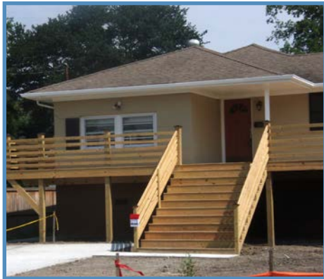
Norfolk has elevated several homes with funds from the Hazard Mitigation Assistance Grant Program to prevent future flooding.
