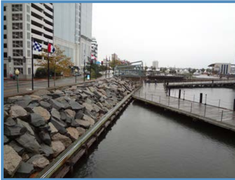
Norfolk's downtown is protected by a floodwall and several gates. Floodgates and walls can provide protection while becoming part of a natural urban landscape.
