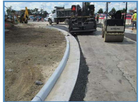
In order to reduce flooding, a section of westbound Brambleton Avenue between Colley Avenue and the Brambleton Bridge has been widened and elevated. The increase in elevation has decreased the impact of flooding during high tide events which has improved access to the region's medical complex.
