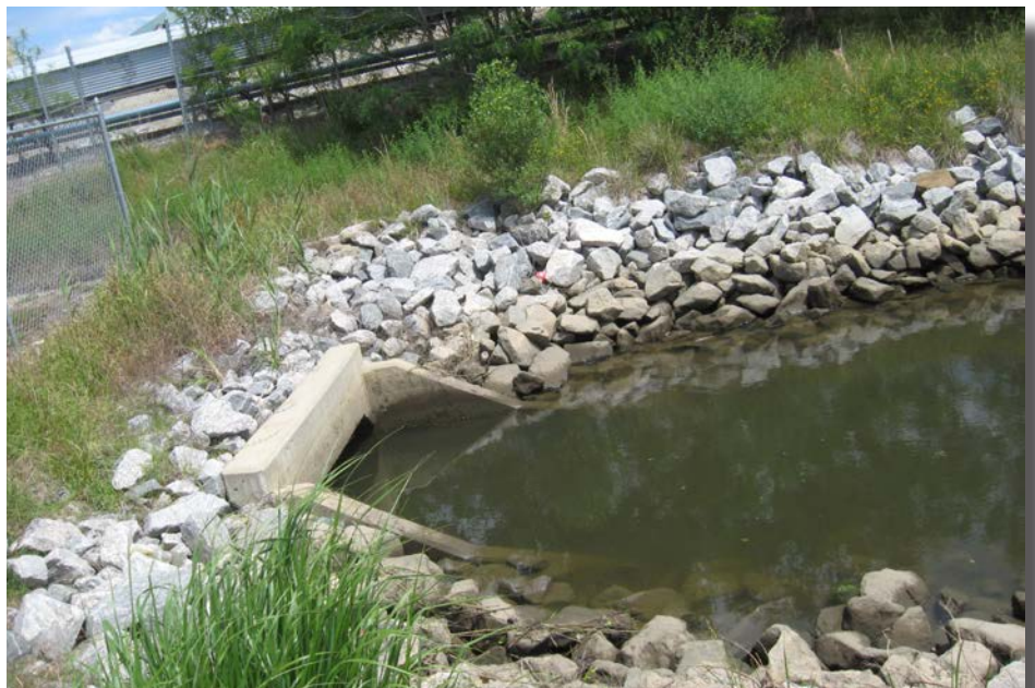
Stormwater culverts manage the flow of water from roadways and neighborhoods.
