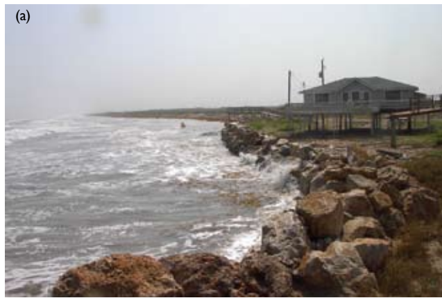
Figure 6.3 Two types of stone revetments (a) near Surfside, Texas and (b) at Jamestown, Virginia [Photo source: ©James G. Titus, used with permission].
