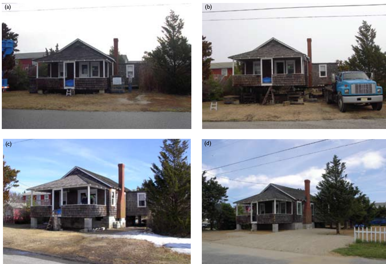
Figure 12.5 Elevating land and house. (a) Initial elevation of house in Brant Beach, New Jersey. (b) Structural beams placed under house, which is lifted approximately 1.5 meters by hydraulic jack in blue truck. (c) Three course of cinder blocks added then house set down onto the blocks. (d) Soil and gravel brought in to elevate land surface (January through June 2005) [Photo source: ©James G. Titus, used with permission].
