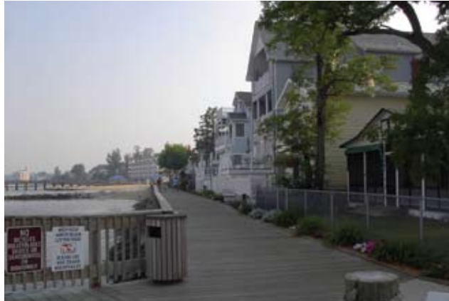
Figure 8.7 Public access along a bulkheaded shore. In North Beach, Maryland, one block of Atlantic Avenue, is a walkway along Chesapeake Bay (May 2006) [Photo source: ©James G. Titus, used with permission].
