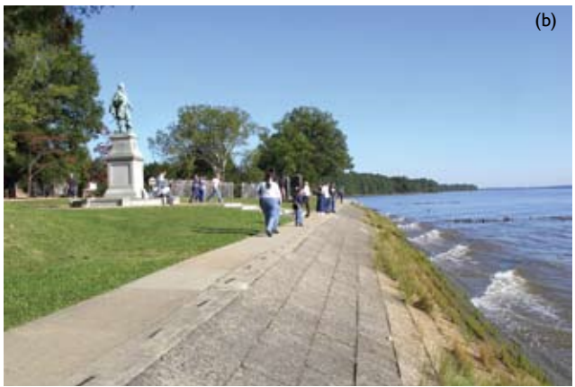
Figure 6.3 Two types of stone revetments (a) near Surfside, Texas and (b) at Jamestown, Virginia [Photo source: ©James G. Titus, used with permission].
