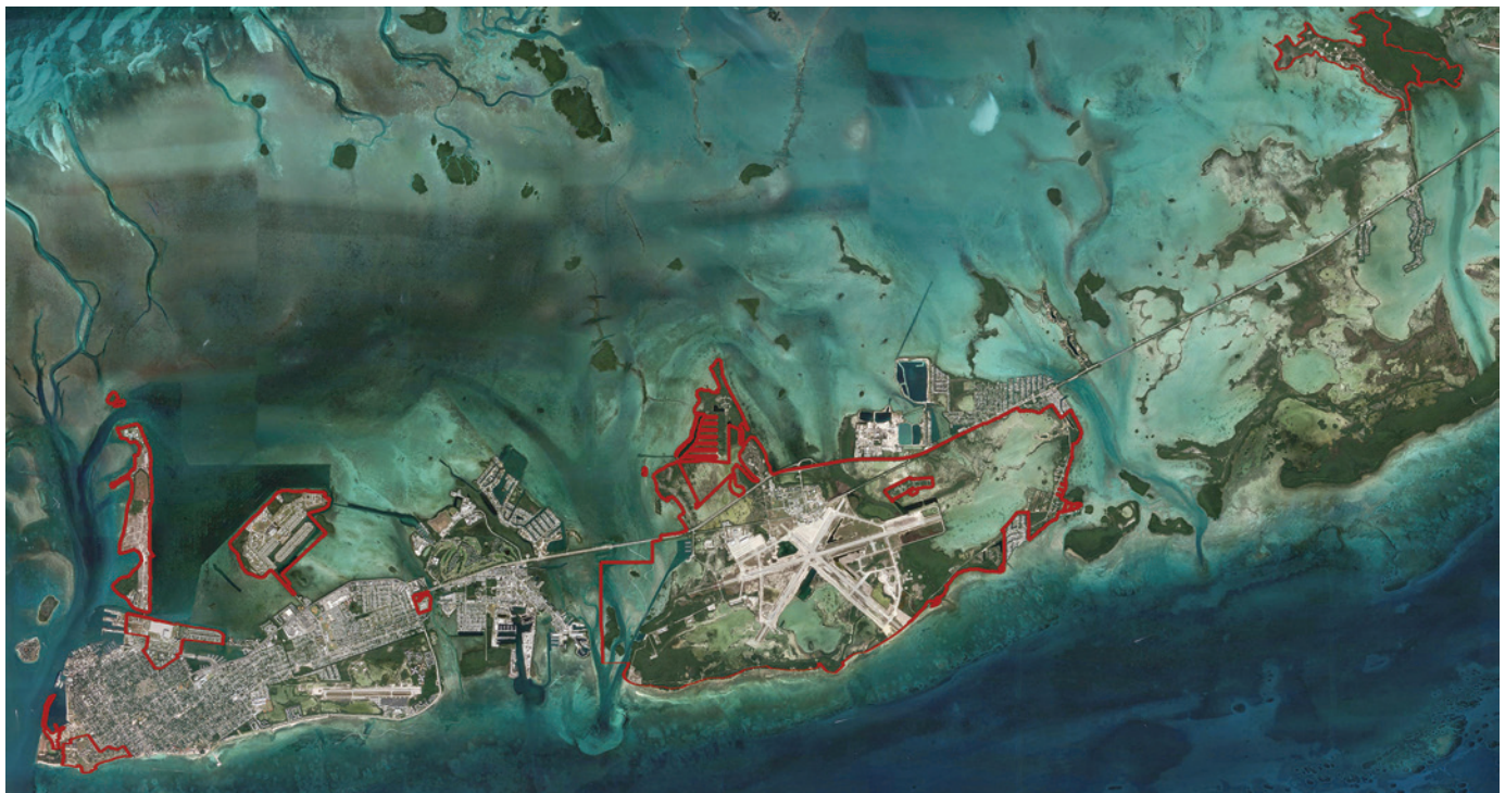
The projected reach of future daily high tides, shown in the top panel, encompasses currently utilized land at NAS Key West, shown in the bottom panel. The highest scenario is mapped here.
