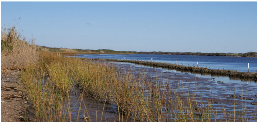
FIGURE 3-6 Nature-based approaches to erosion control in Mobile, Alabama. The oyster reef is seaward of the marsh edge.
