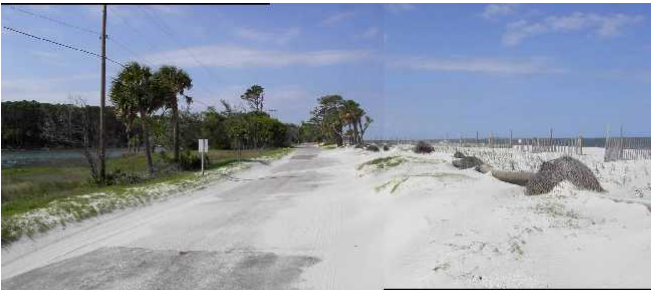
Photo 32. Evidence of Overwash on Hunting Island. Park authorities installed dune fencing in hopes of protecting the road at a narrow portion of Hunting Island. Nevertheless, storms and winds appear to be causing a small dune to form on top of the marsh on the landward side of the road
