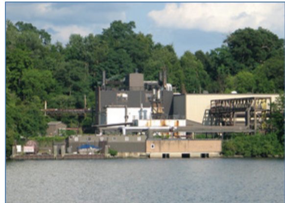
Sea level rise will push the Hudson River salt front upriver, threatening water supplies of several Hudson Valley communities and businesses, including this water intake at the IBM facility in Poughkeepsie.
