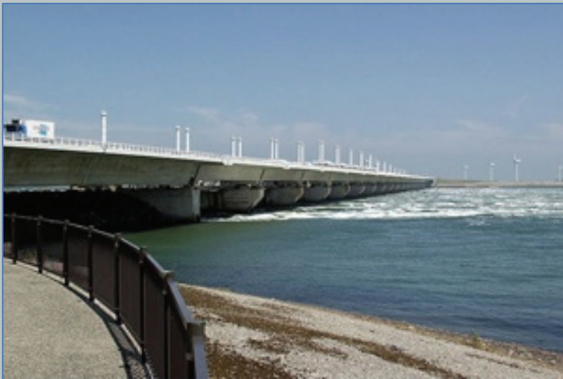
Eastern Scheldt storm-surge barrier, Netherlands. Credit: Raimond Spekking/ Wikimedia Commons/CC-NY-SA-3.0 & GFDL
