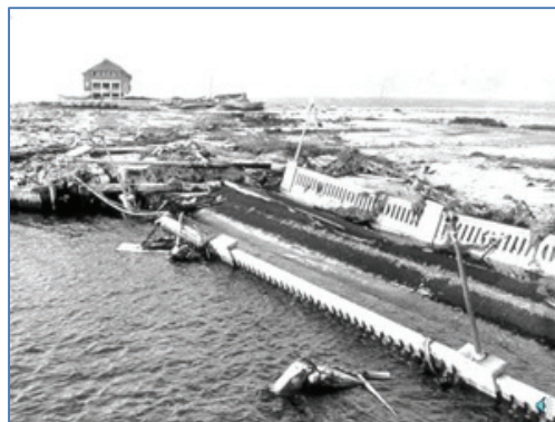
Only a small, sagging portion of the main building of the West Bay Beach Club in Quantuck, Suffolk County, remained after the 1938 "Long Island Express" hurricane.
