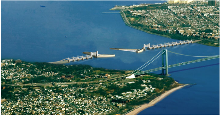
Fig. 12 Conceptual design of a storm surge barrier in NYC. Source: Aerts et al. (2009)
