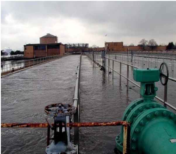
Fig. 8 Photo of treatment tanks overflowing at a Bronx WPCP during March 2001 storm
