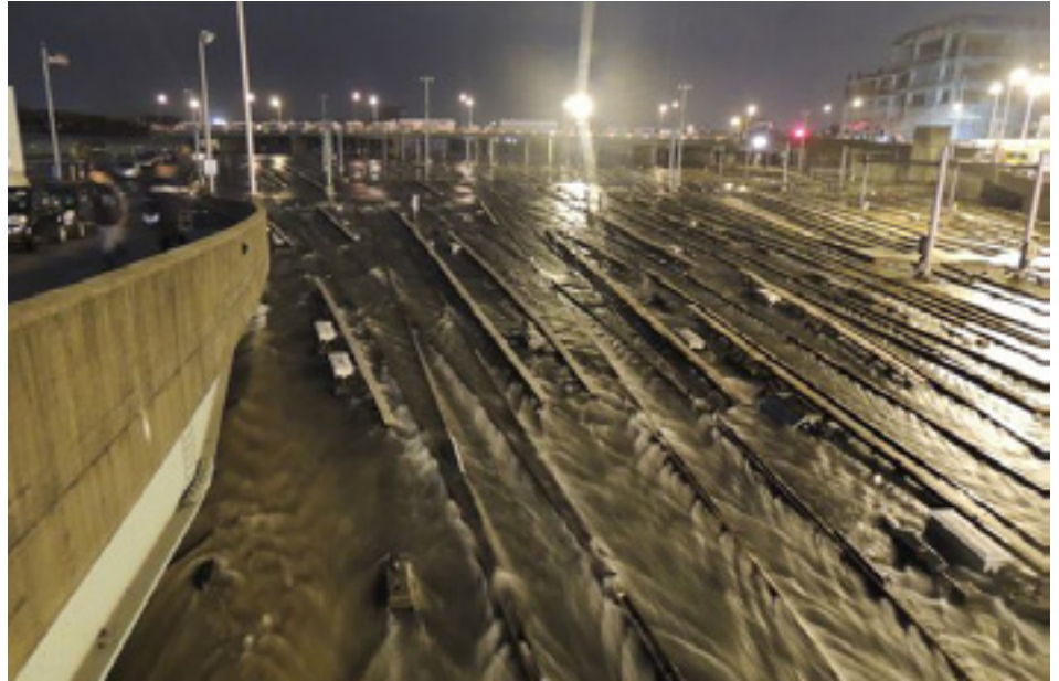
Figure T-13: Floodwater inundating LIRR's West Side Yard. All trains had been removed prior to the arrival of the storm. (MTA Long Island Rail Road, 2012)
