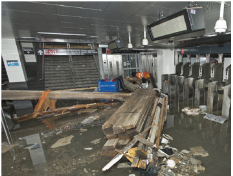
Figure T-12: Damage and debris in the South Ferry subway station following Superstorm Sandy. (MTA, Patrick Cashin, 2012)
