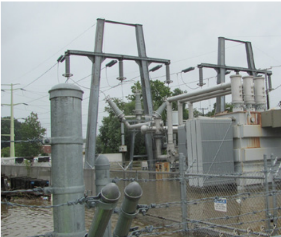
Figure E-04: Flooded substation (Flickr, FirstEnergy Corp, 2012)
