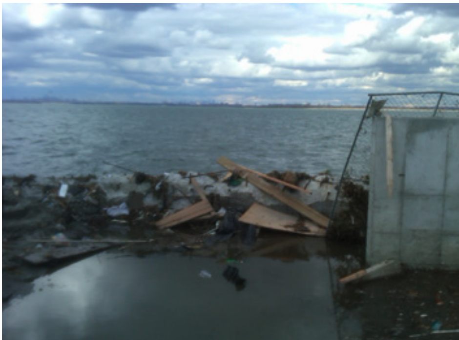
Figure L-07: Thick iron reinforced seawall in the Rockaways broken by force of storm surge (NYSDEC, 2012)
