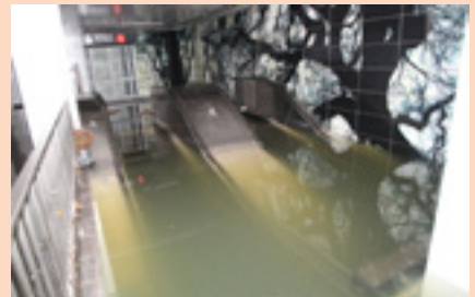
Figure T-03: Escalators under water at the South Ferry subway station. (MTA, 2012)
