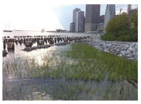
"Soft edges" deployed at Brooklyn Bridge Park are part of the site's stormwater management system. The constructed wetland also dissipates wakes and provides habitat.
