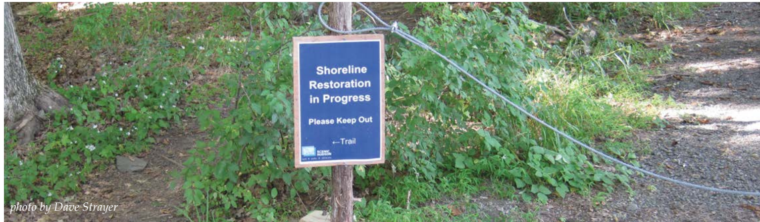
Using signs, barriers, and a new path to direct people away from an eroding shoreline.
