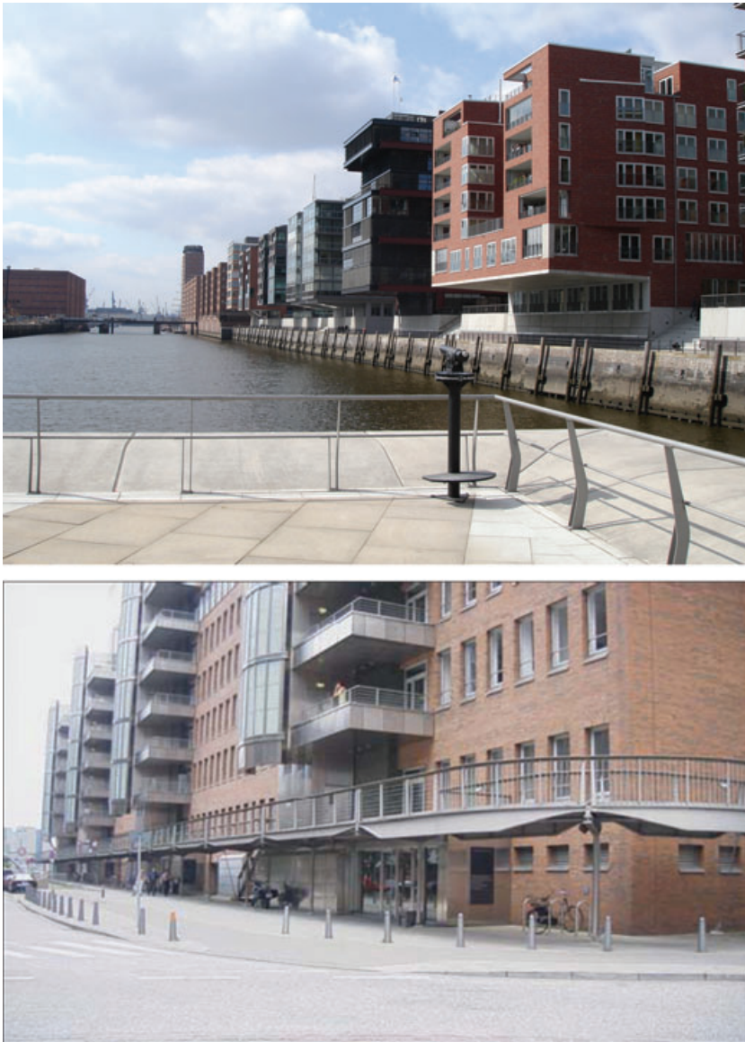
Figure 7.2. HafenCity (City of Hamburg, Germany) with the boardwalk at about 9 ft and the residential apartments at a level of 22 ft (top). Emergency serveway above the design water level at HafenCity (bottom). Source: Jeroen Aerts.
