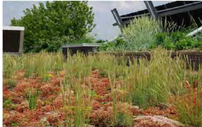
Rancho Verde site green roof
