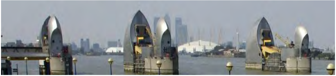
Image of the Thames Barrier 49
