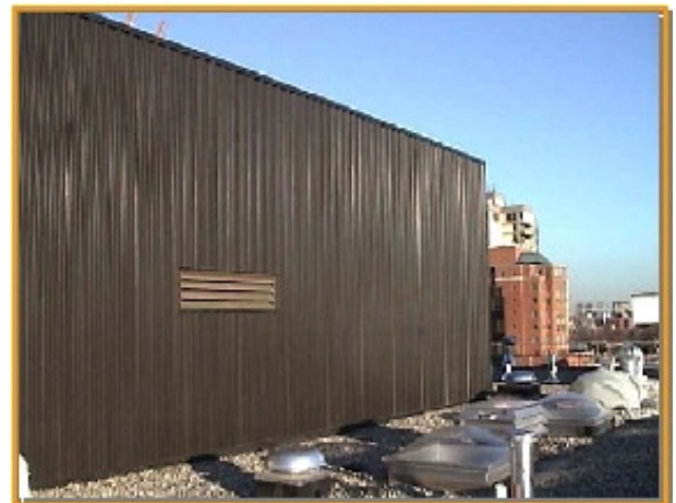
Solar Air Heating System on the Roof of Houghton Place Apts. in Cambridge, MA
