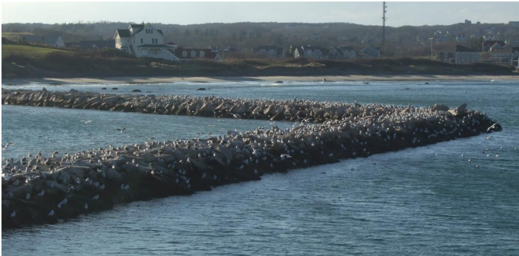
North and west sections of Old Harbor Breakwater
