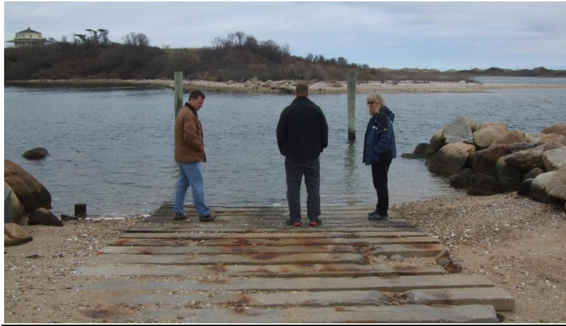
Boat ramp at New Harbor
