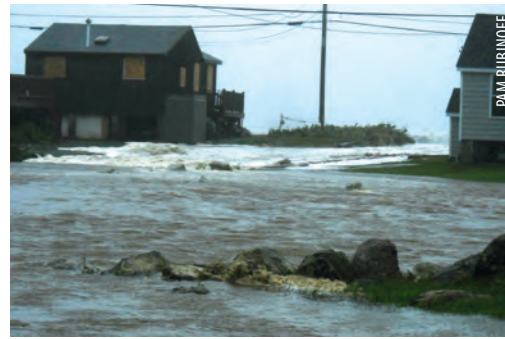
Flooding, such as in Matunuck during Tropical Storm Irene, is on the rise.
