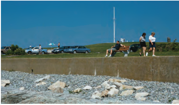
Beaches will be more vulnerable to erosion; previous efforts to stabilize them with seawalls and revetments have often led to even greater erosion.
