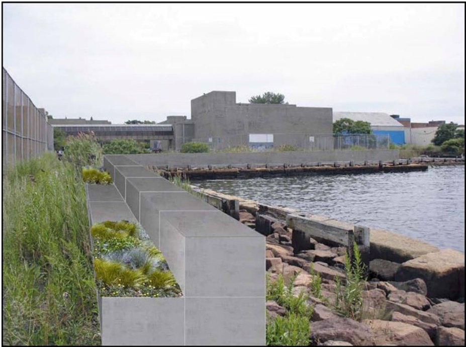
Fig. 2 Conceptual modular sea wall design protection for a school and community center in East Boston (Figure created by Woods Hool Group, Inc, E. Falmouth, MA. used with permission)
